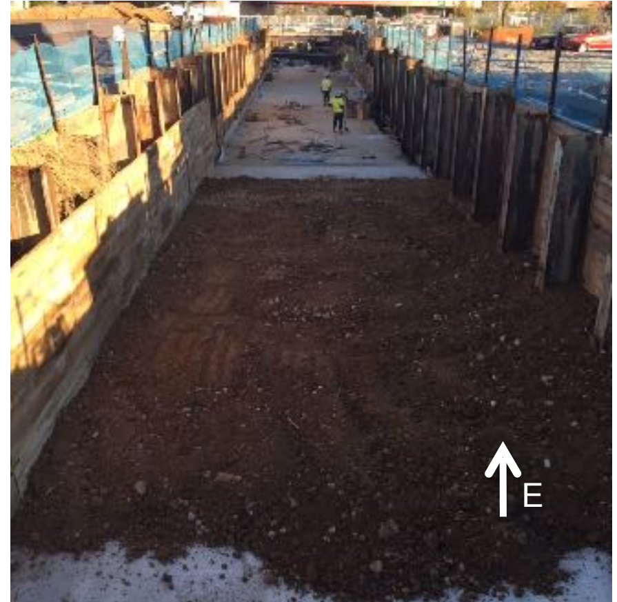
Backfilling Has Started
