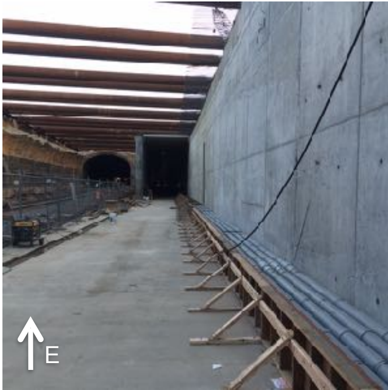
Invert and Walls Complete Precast Roof Soffits Installed
