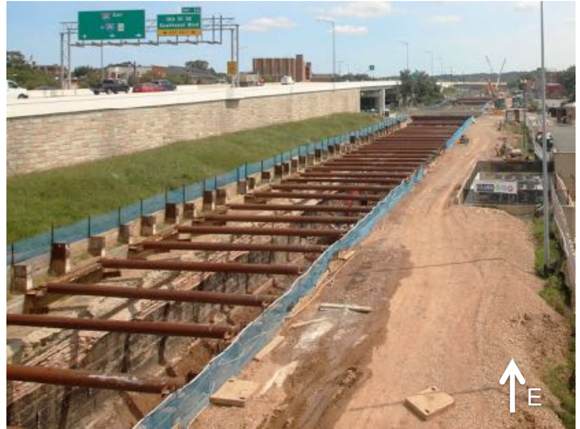
Tunnel Demolition and Excavation
