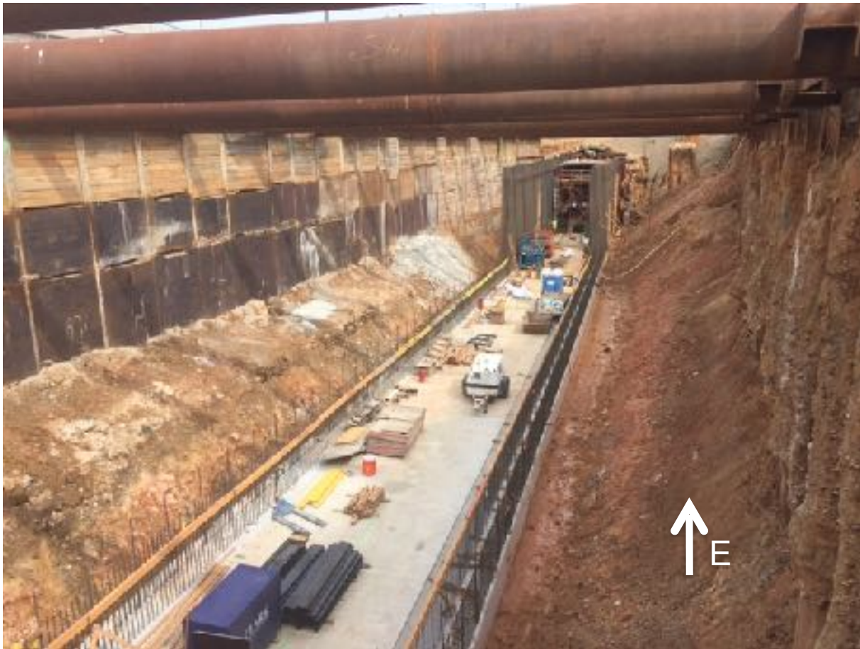
Tunnel Inverts and Walls
