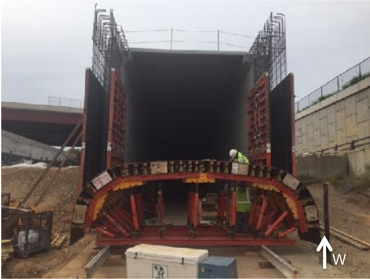
Forming Tunnel Portal
