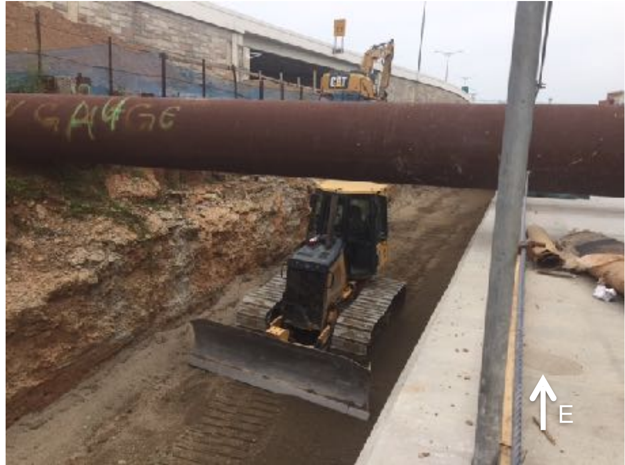
Backfilling to Final Grade
