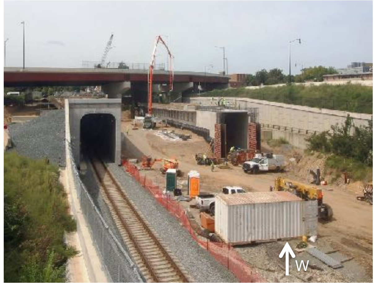
Pouring Concrete Roofs
