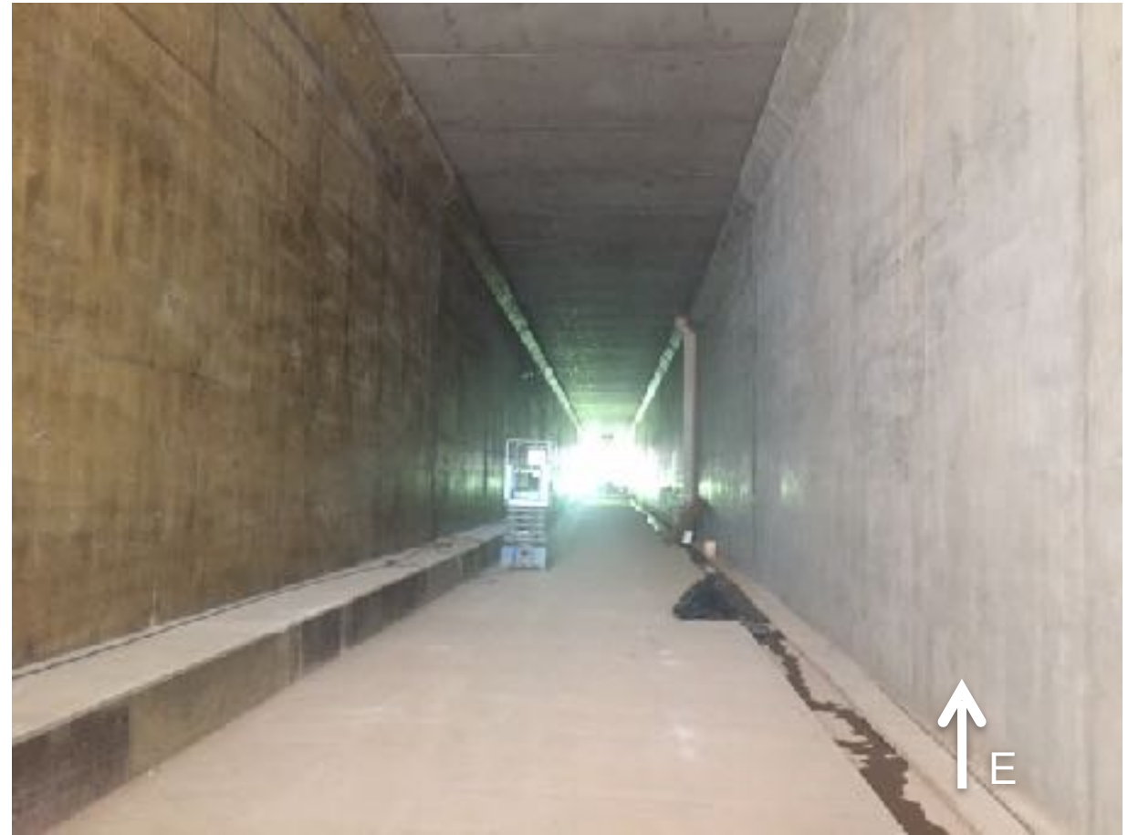
Inside the Tunnel
