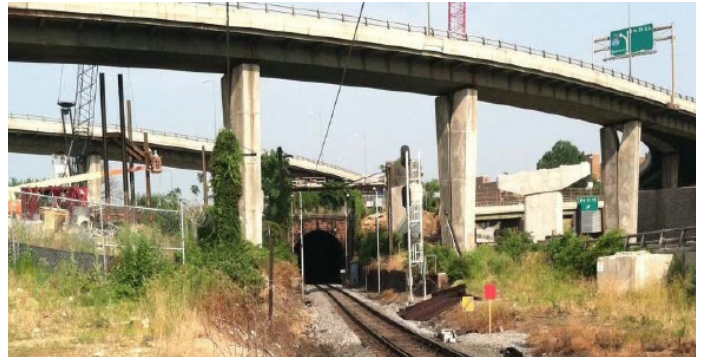
A view of the east portal of the Tunnel
