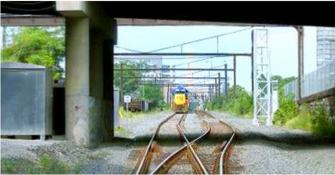
Looking west from the Virginia Avenue Tunnel portal near Garfield Park
